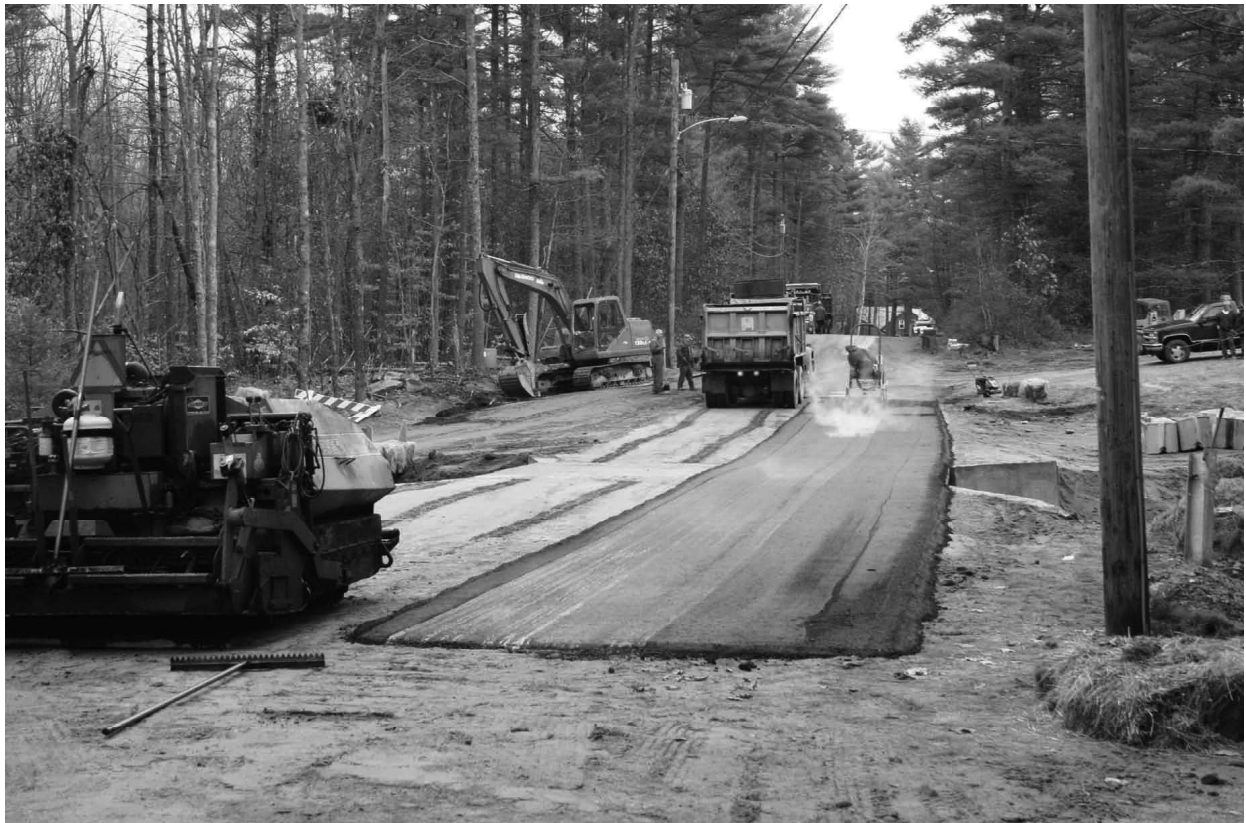
On Monday, November 26, 2007 Southern Maine Paving arrived to pave the bridge and the approaches. After the paving was completed, the guardrails were attached to the new bridge. These guardrails were extended beyond the two abutments. The guardrails and the deck were removed from the temporary bridge. The approaches to the temporary bridge were excavated down to the original ground level.
