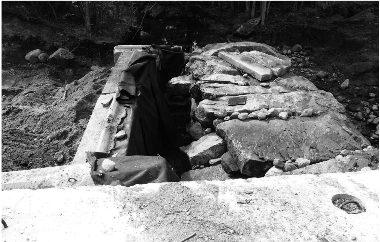
This is the down stream end of the culvert on Jenkins Brook at the Lower Tarbox Road. A geotextile fabric was used to cover the form before the concrete wall was poured. Notice the smaller rocks at all the granite joints to hold back the wet concrete.
