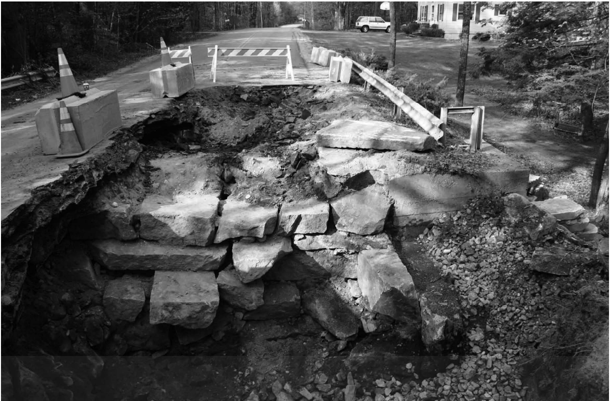
The outside of the culverts are very uneven. Building traditional wood forms would have been very costly. Using large precast concrete interlocking blocks like the ones at the top left provided forms that allowed excavation, forming and pouring each day.
