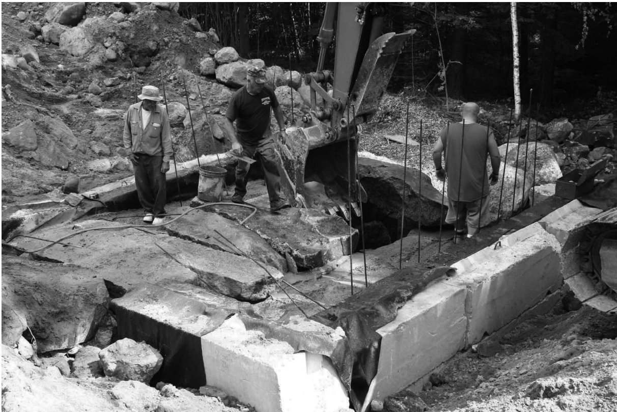
This is the top or roof of the Muddy Brook Culvert. Ken Stone is carefully placing the granites under the direction of Alton (Whitey) Meserve, center. To the left is former Hollis Road Commissioner Robert (Bob) Hanson. To the right is Ryan Stuart.
