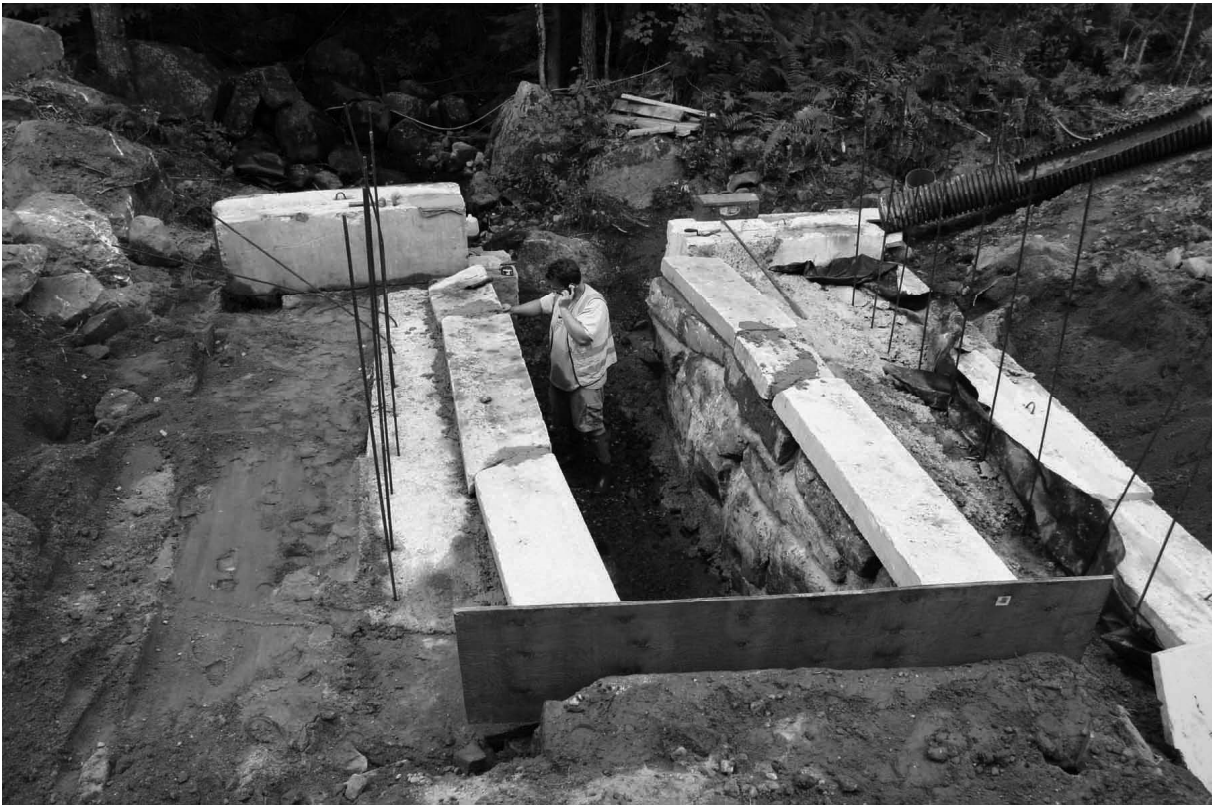
Above is the inlet to the Muddy Brook culvert on Deer Wander Road. The whole culvert had to be rebuilt from the bottom up and widened. The height was also increased to give it more capacity. Rob Hanson is directing operations from inside the culvert.
