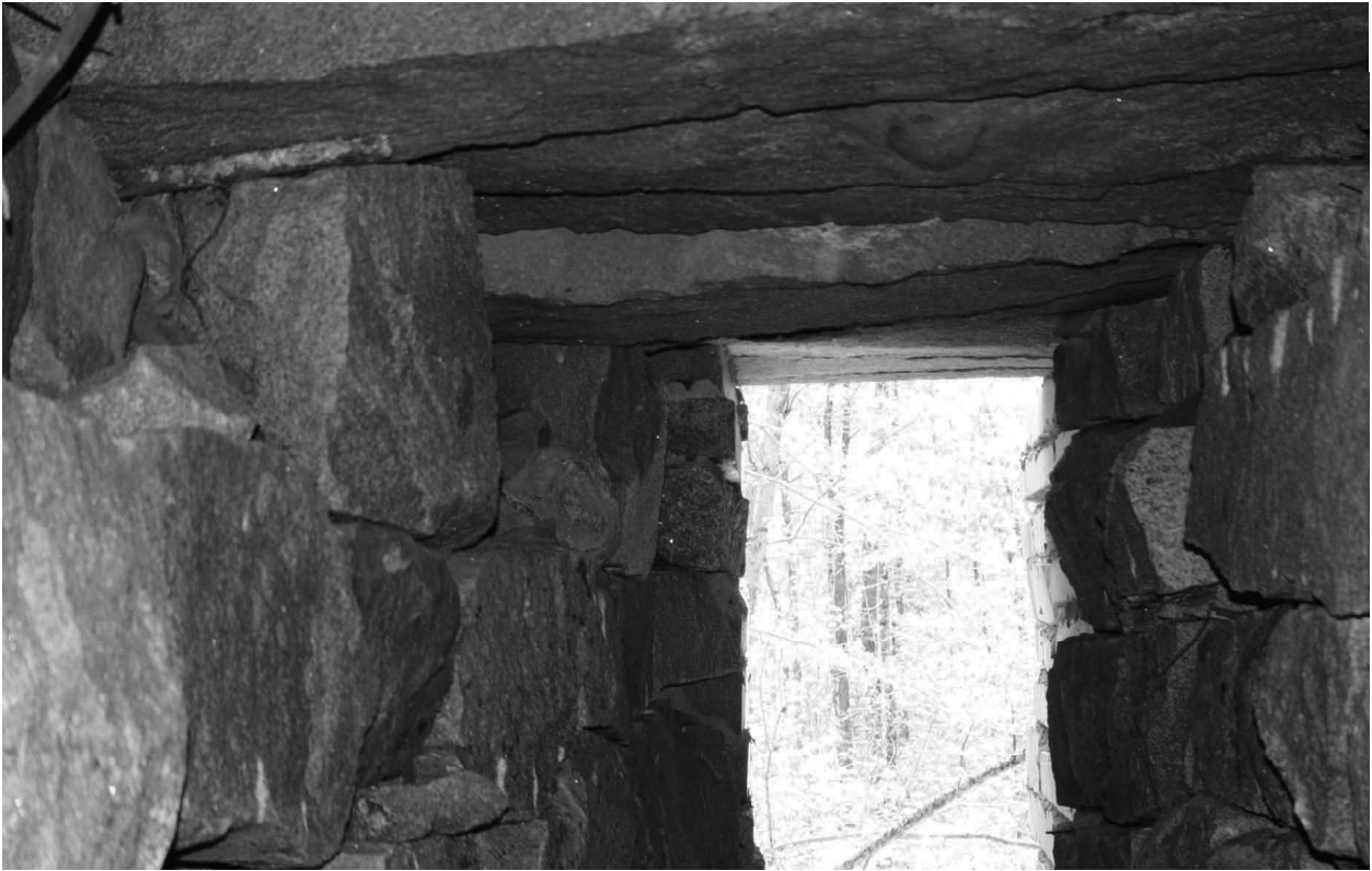
The above photo is inside the Haley Road culvert looking down stream. The stones that stick out into the opening tend to catch and redirect the water left and right from the course of the culvert, sending water behind the granite blocks causing wash outs.
