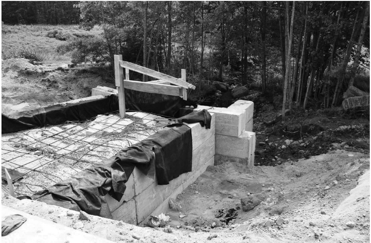
Each time a wall was poured, reinforcing rod was inserted into the pour. Once the concrete set up, the rods were bent from one side towards the other and tied. More reinforcing rod was installed in line with the culvert and tied before the top was poured.
