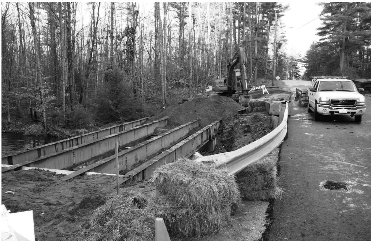
On Monday, November 26, 2007 Southern Maine Paving arrived to pave the bridge and the approaches. After the paving was completed, the guardrails were attached to the new bridge. These guardrails were extended beyond the two abutments. The guardrails and the deck were removed from the temporary bridge. The approaches to the temporary bridge were excavated down to the original ground level.
